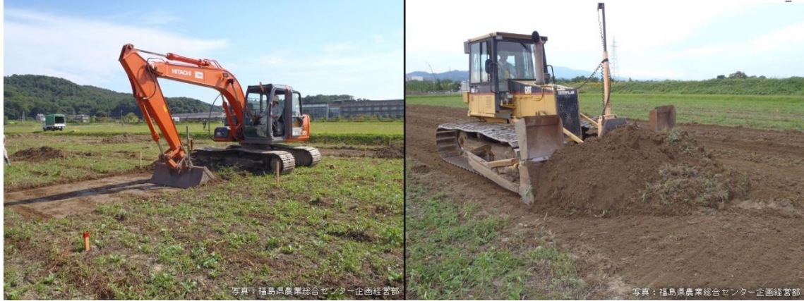
Fig.1-2 Photos of topsoil scraping procedures [14].
